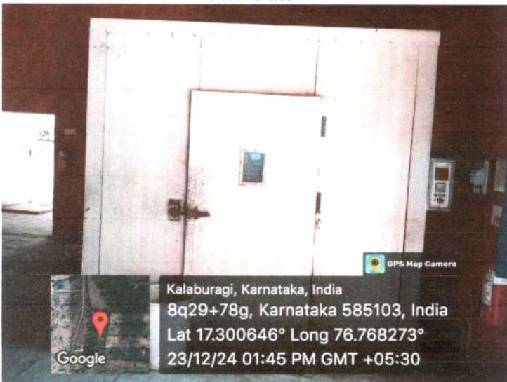
Cold storage room
