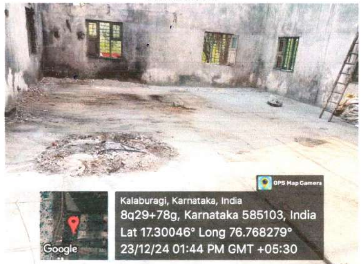
Old incineration room
