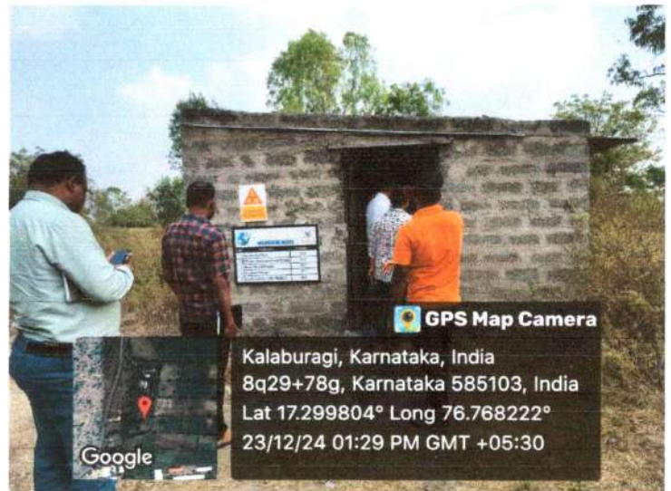
Hazardous waste storage room
