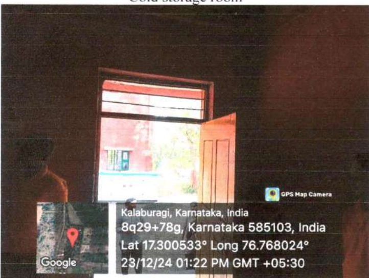
Ventilation for untreated storage room
