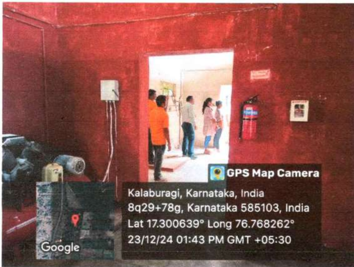
Fire extinguisher and First aid kit
