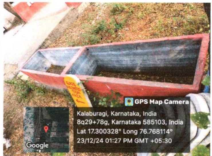
Glass disinfection pit
